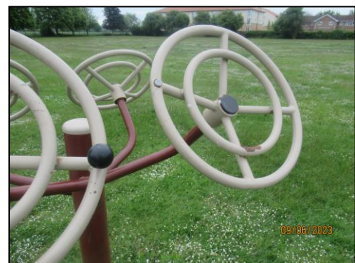
(Missing hand holds at hand wheels – library photo)
